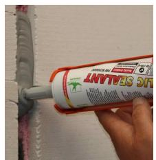
2. Apply FP Acrylic Sealant to the cured FP PU Foam and make sure the joint is completely filled with material.
