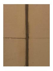
4. The joint is now fire retardant and securely sealed with FP PU Foam and FP Acrylic Sealant.
