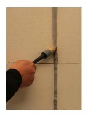
3. Finish the joint with a brush, moistened with water.
