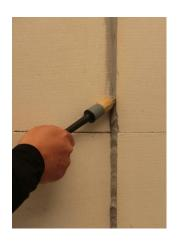
4. Finish the joint with a brush, moistened with water.
