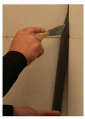
2. Place backer rod at the right depth. Joint width/3 + 6 mm = joint depth Example: 15mm/3 = 5+6mm = 11mm depth
