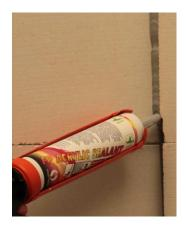
3. Apply FP Acrylic Sealant to the backer rod and make sure the joint is completely filled with material.
