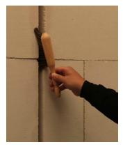
Clean from dust with a soft brush and remove loose particles. When needed pre-treat the joints with a primer for porous substrates.
