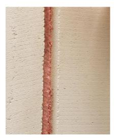
1. See application guidelines for FP PU Foam to apply the foam recessed, with result as beside picture.
