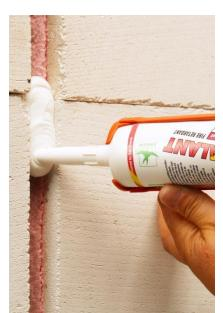
2. Apply FP Hybrid Sealant to the cured FP PU Foam and make sure the joint is completely filled with material.
