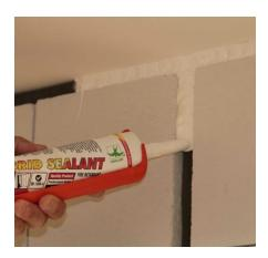
3. Apply FP Hybrid Sealant to the backer rod and make sure the joint is completely filled with material.
