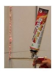
4. Fill the complete depth of the joint with FP PU Foam. Place the tip of the gun or adaptor as deep as possible in the joint, and fill full depth of the joint with with FP PU Foam.
