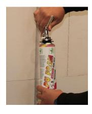
3. Rotate the gun or hand-adaptor on top of the foam cannister. Alsways keep the bottle upright when fastening the gun or adapter. Shake cannister at least 20 times in a vertical direction.
