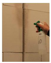
1. Pre-moisten the joint with water by for example using a spray bottle.
