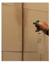
2. Pre-moisten the joint with water by for example using a spray bottle.
