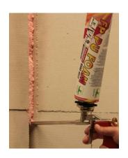
3. Fill the joint a bit recessed, the foam will expand further.
