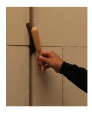
1. Clean from dust with a soft brush and remove loose particles.
