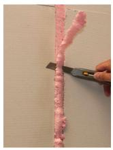
5. Cut off the surplus of cure foam with a sharp knife after about 1 hour.
