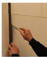
4. Place the PE backer rod at the right depth, so the foam is blocked an cannot further expand outwards. This process creates the right depth for the FP Sealant.
