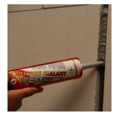
3. Apply FP Silicone Sealant to the backer rod and make sure the joint is completely filled with material.
