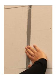
4. The joint is now fire retardant and securely sealed with FP PU Foam and FP Silicone Sealant.
