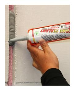
2. Apply FP Silicone Sealant to the cured FP PU Foam and make sure the joint is completely filled with material.
