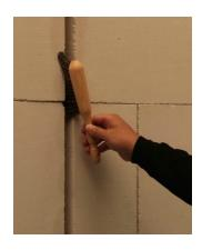
1. Clean from dust with a soft brush and remove loose particles. When needed pre-treat the joints with a primer for porous substrates.
